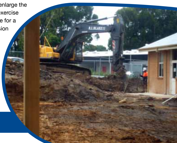
Site clearing is well underway the building
